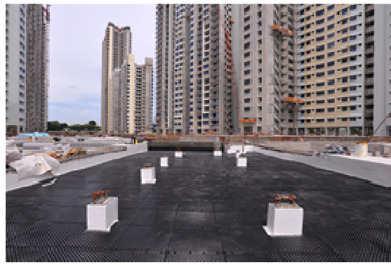
2h) Panels cut to fit plinths.
