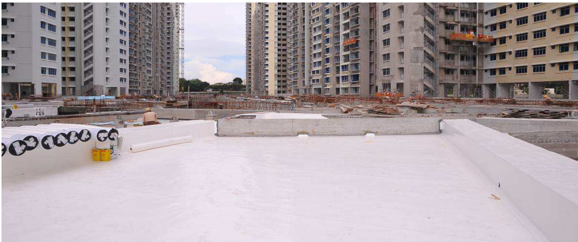
2b) Root-resistant waterproof membrane
