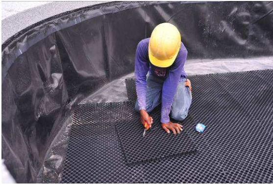
2g) Cut panels to size or fit
