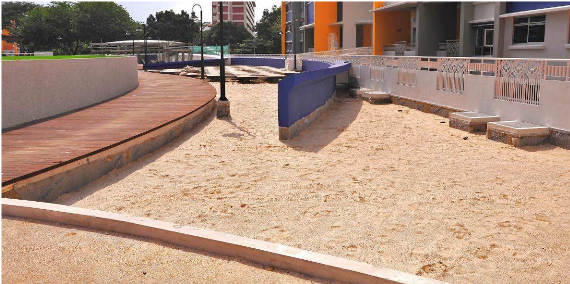
2i) Coarse sand placement awaiting soil
