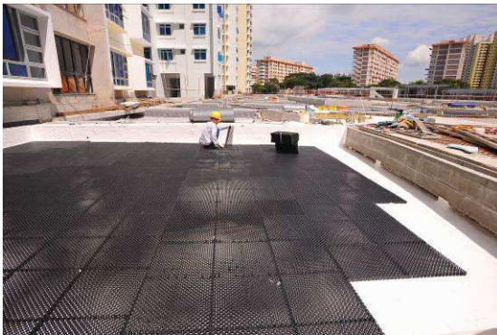
2e) Modules placed directly over waterproofing membrane
